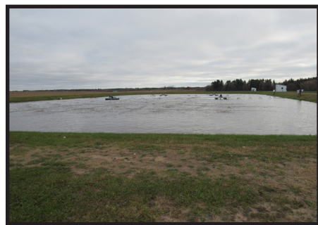
Ponds everywhere. The ponds do a lot of work to help clean waste water in our area. The plant presently treats a combined total of 500,000 gallons per day.
